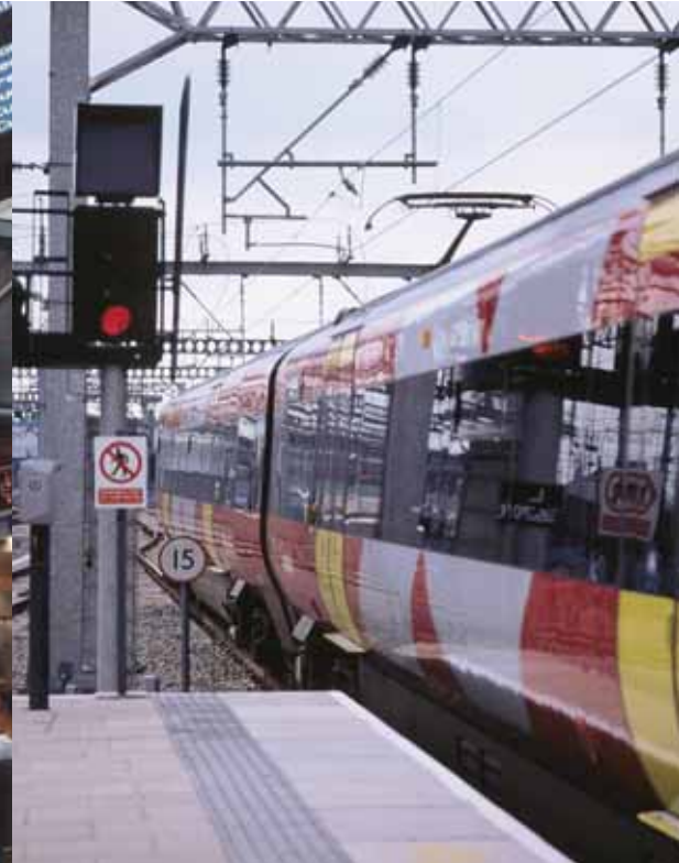
Above: Effective security measures are required to protect people, assets and infrastructure
